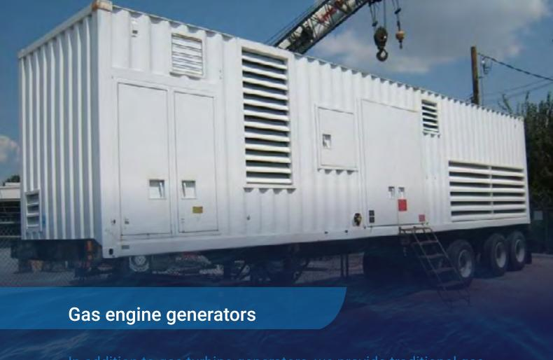
In addition to gas turbine generators, we provide traditional gas engine generators from 500kW to 3.5MW, powered by renowned Waukesha and Caterpillar brands. These traditional generators generally require lower capital investment, but require more preventative maintenance than a turbine that can result in higher operating costs.
