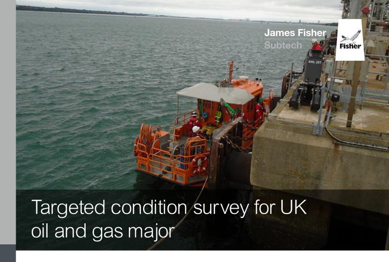
Utilising James Fisher Subtech's (JF Subtech's) air diving capability and remotely operated vehicle (ROV), the team successfully inspected the entire underwater marine jetty infrastructure and completed a targeted condition survey to closely inspect structural condition of piles, jetty legs and associated structures in a busy tidal estuary.
