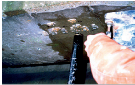
Small diameter coring
