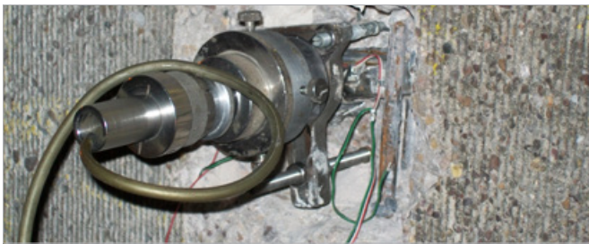
Pre-stressing wires – centre hole method
