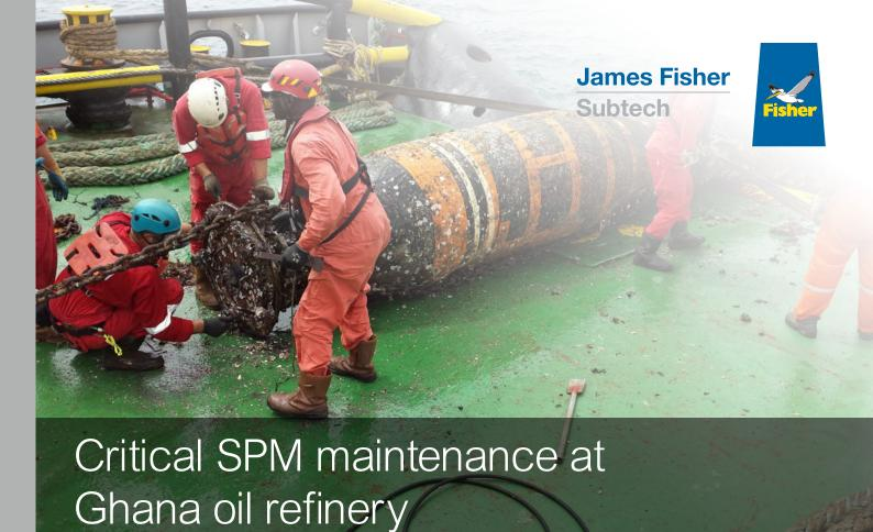
Provision of air diving personnel and equipment in support of inspection and maintenance of customer-owned SPM and relating facilities. Additional support for tanker mooring operations and general field support as required by the customer.
