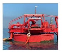
JF Strainstall was contracted by Orwell Offshore to provide a CALM buoy monitoring package to be retrofitted to three existing buoys. These systems will improve operational efficiency, monitoring environmental and mooring loads from the tanker and local area, this information is shared wireless to shore-side and with the tanker.
