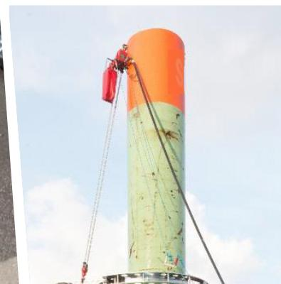
This tool is a remotely operated caisson cleaning system which uses a vertical frame and circular power heads to secure around the caisson. The system is easily deployed to remove marine growth, facilitating inspection and providing an alternative to the more traditional rope access systems. The system also has Electro Hydraulic and Lever operated hydraulic system options.
