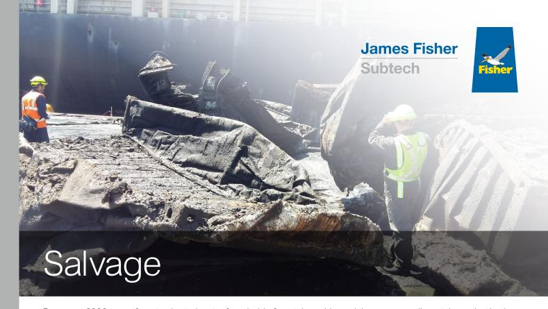
Pump out 6000 tons of contaminated water from hold of container ship and then remove all containers that had been damaged in a chemical explosion and subsequent fire.
